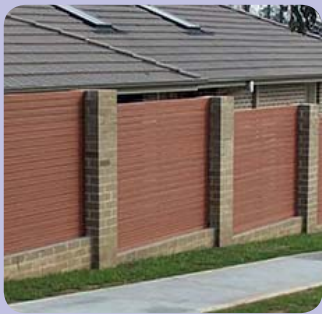
1.8M DWARF WALL WITH HORIZONTAL TIMBER SLATS
